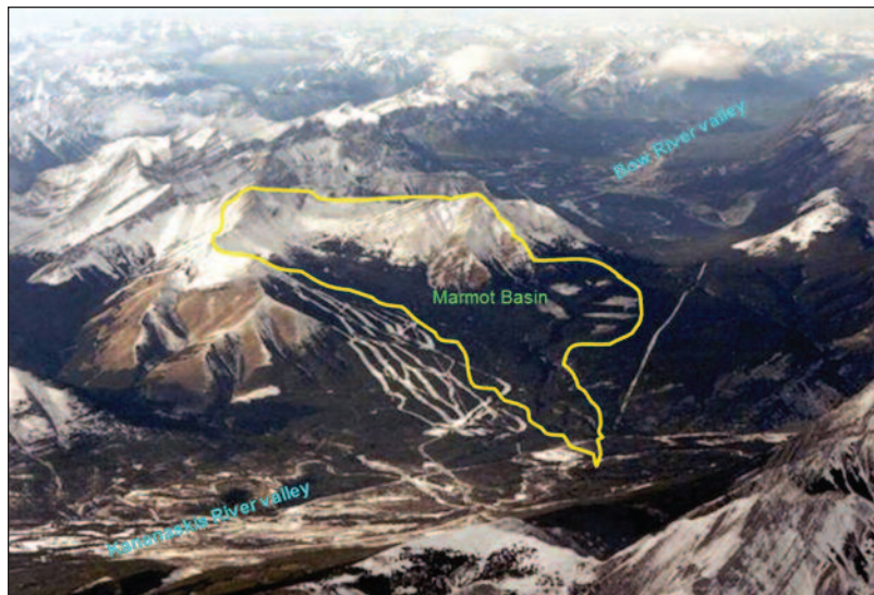
Fig. 1. Aerial view of Marmot Creek Experimental Watershed (Courtesy Centre for Hydrology, University of Saskatchewan)
